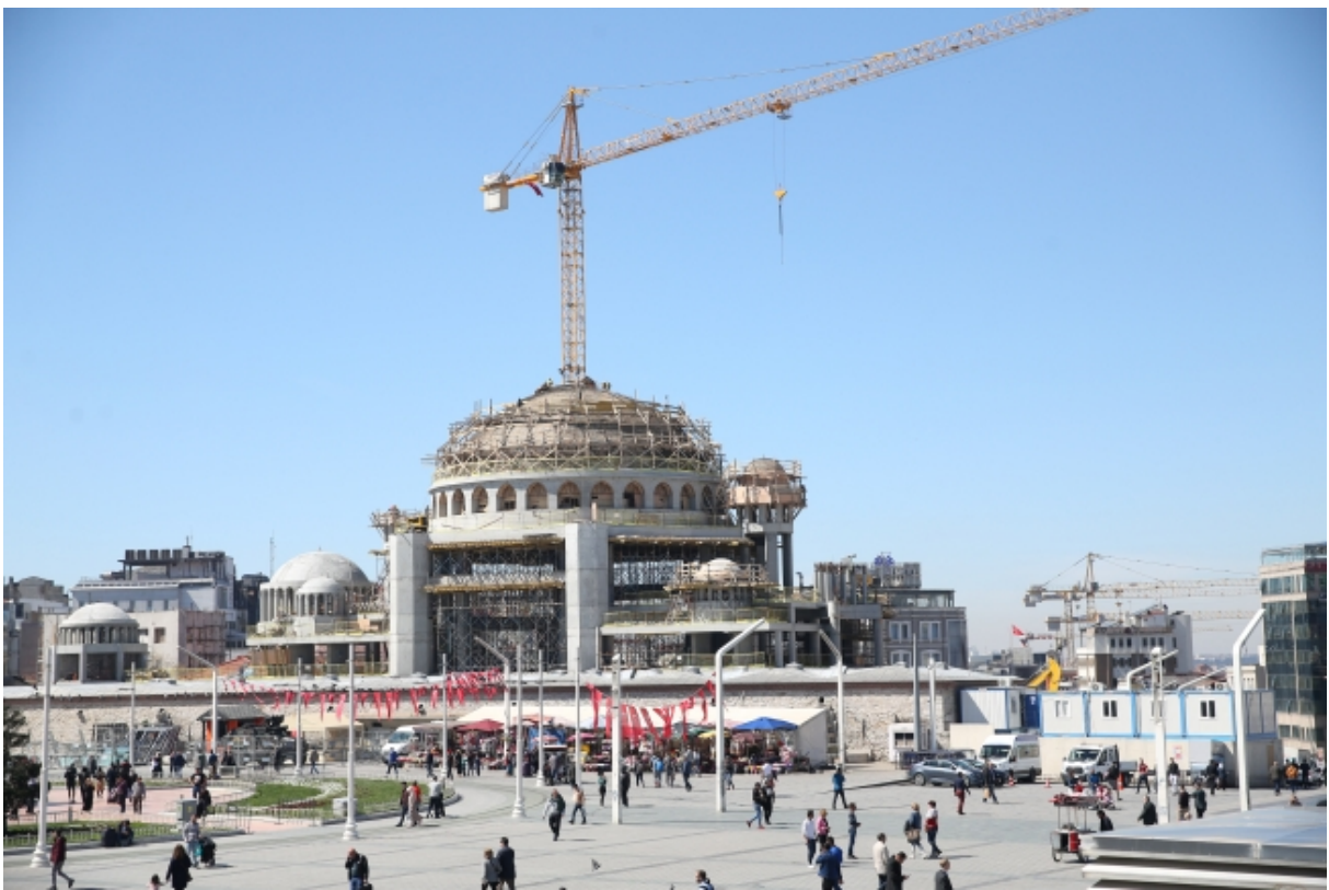
Fig.13 Taksim Square mosque under construction.
